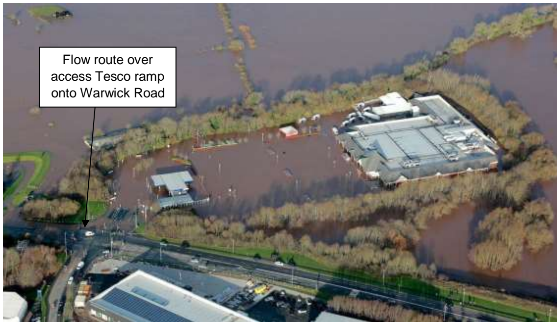
Photograph 1: Flooded Tesco store with the flow route onto Warwick Road visible
