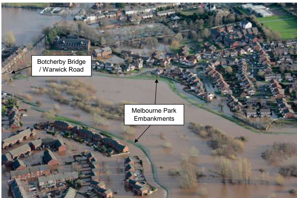
Photograph 2: Melbourne Park and River Petteril during flood event
