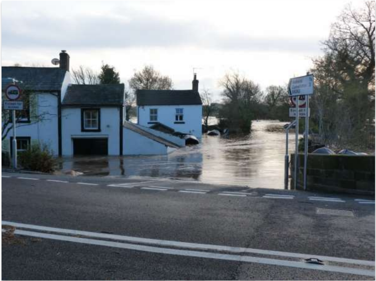
Figure 8: Flooding to Bridge Cottages off the A69
