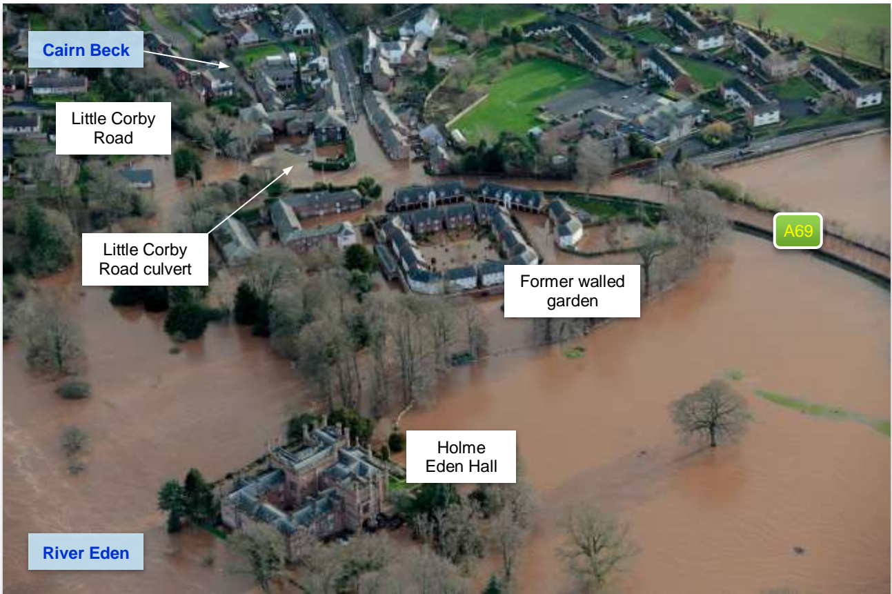
Figure 11: Flooded extents in the centre of Warwick Bridge
