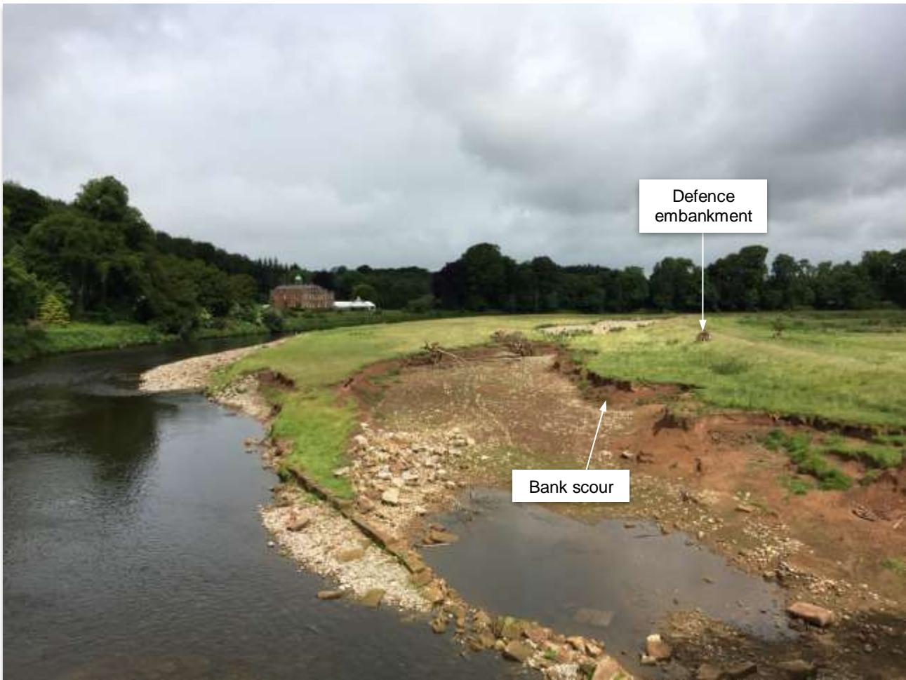
Figure 12: Scouring to right bank of the River Eden downstream of the A69
