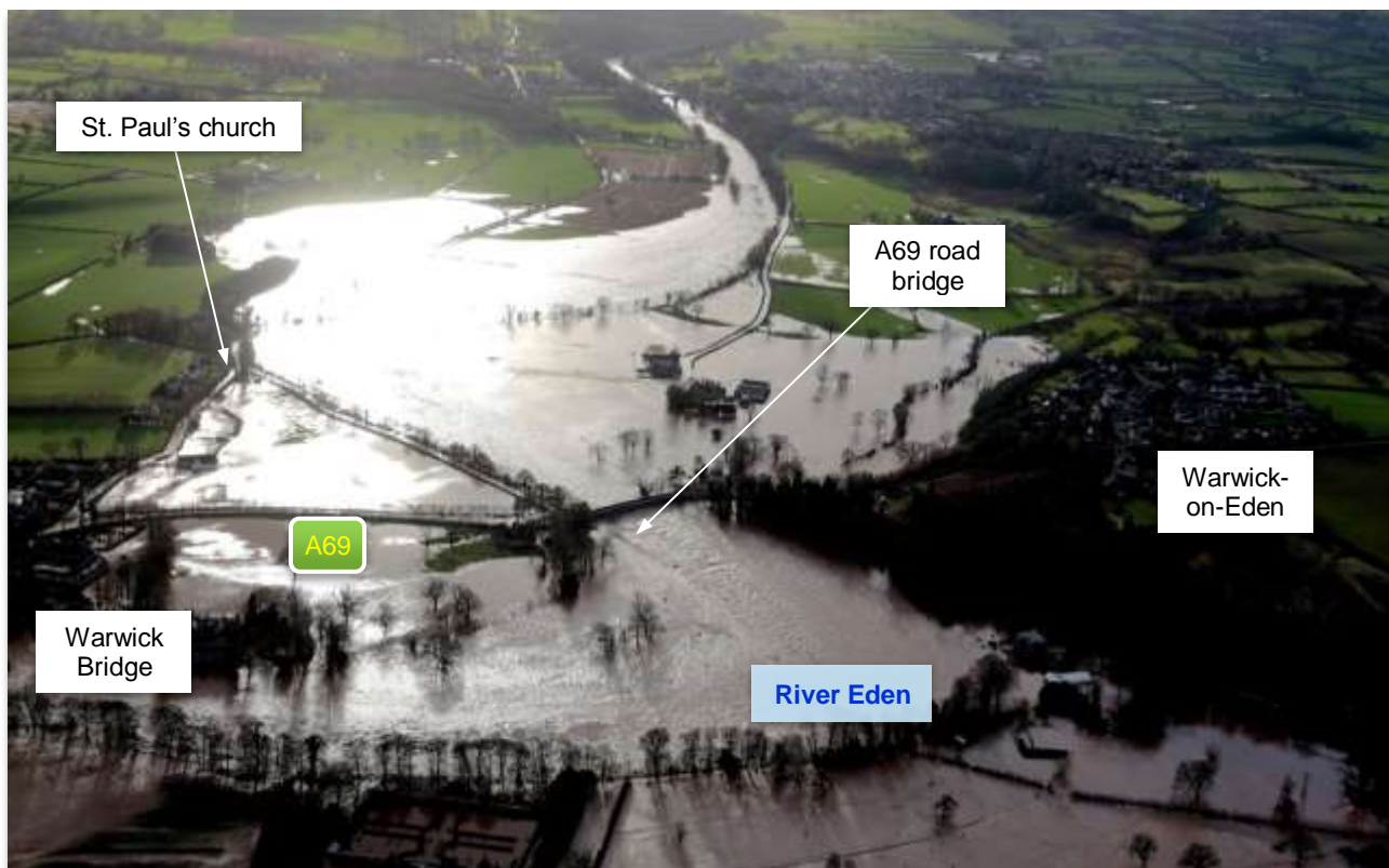
Figure 7: Flooded extents at Warwick Bridge on the 6 th December 2015, looking south
