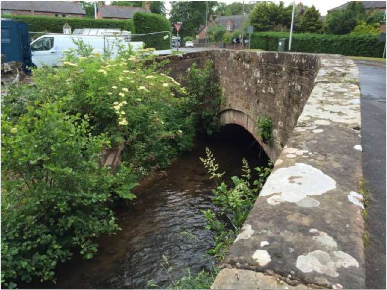
Figure 13: Little Corby Road culvert (Cairn Beck)
