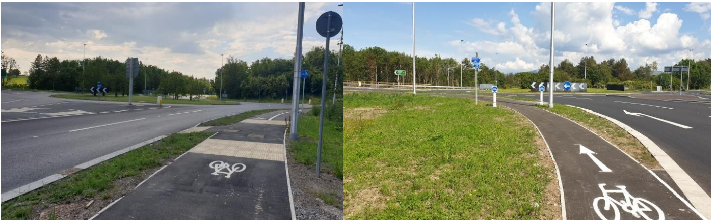
Left: A66/A595 Bridgefoot Roundabout; right: A66/A595 Papcastle Roundabout
