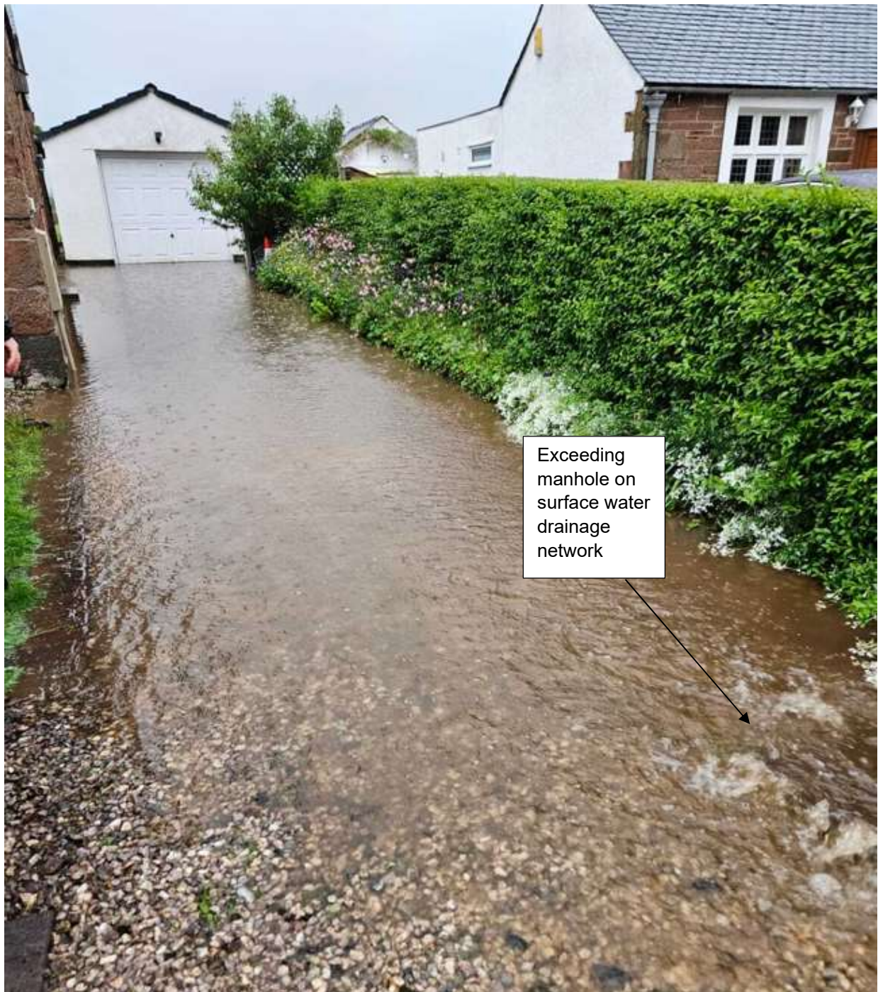
Figure 11. Exceeding manhole in private driveway
