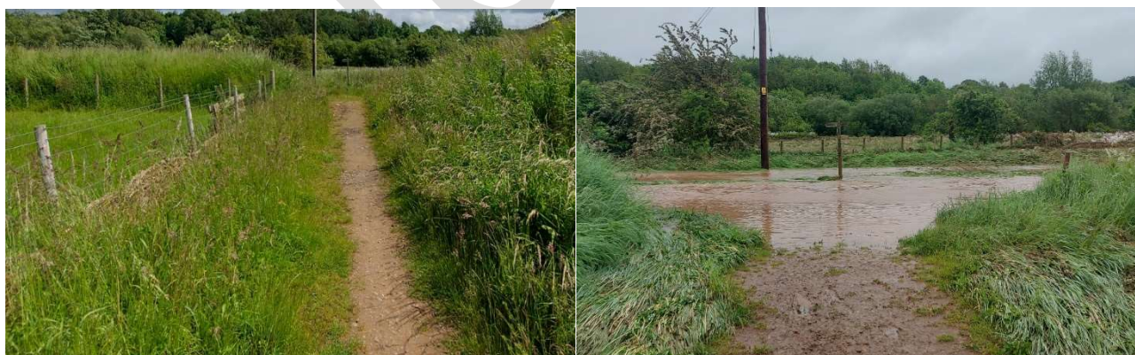
Figure 12: Post flood photograph showing wrack mark on the fence that had carried flood water from the Caldew.
