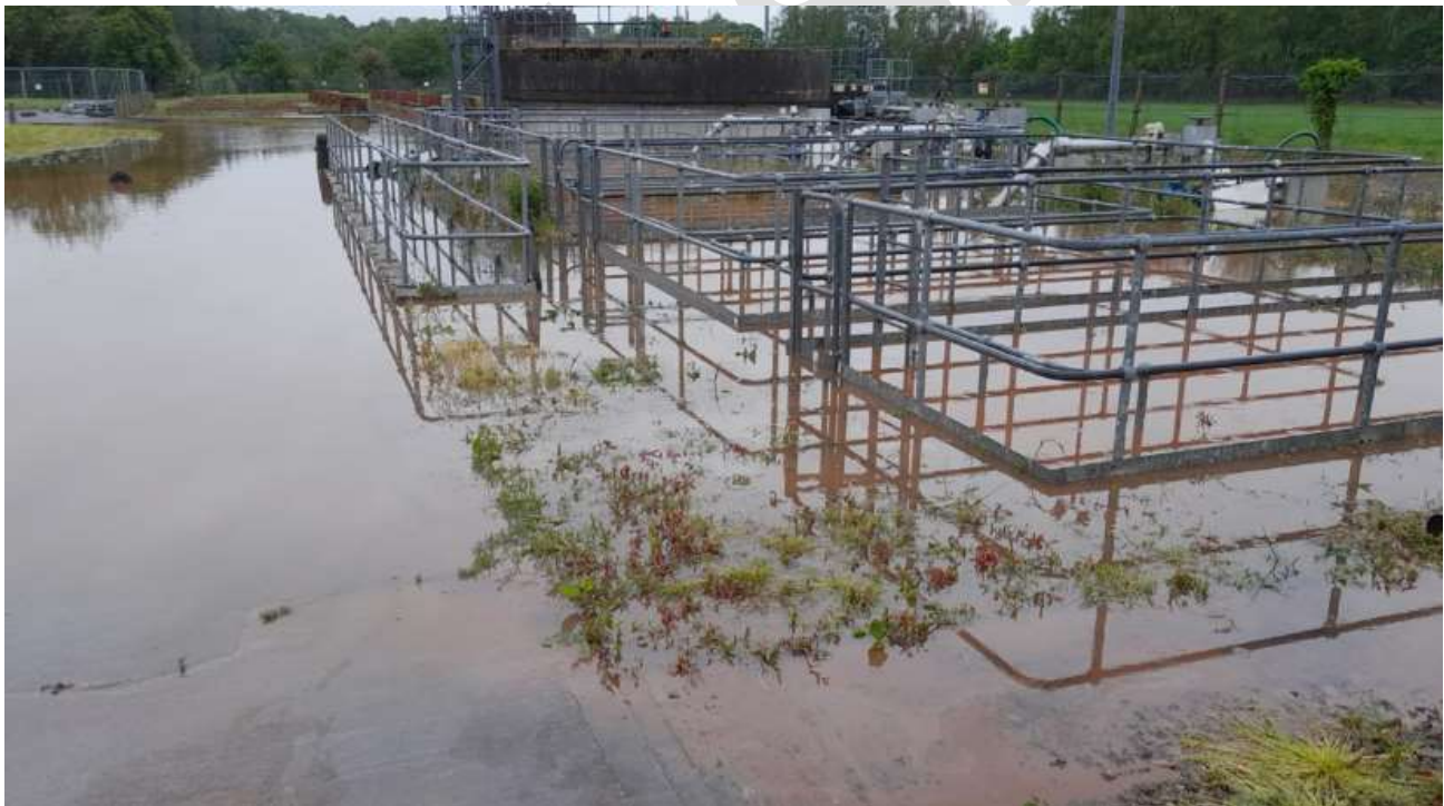
Figure 14: United Utilities treatment works
