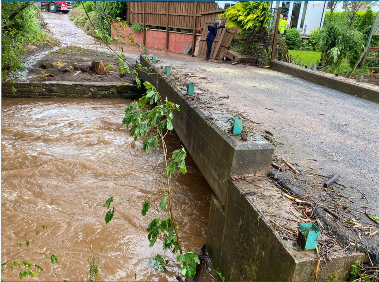
Figure 23: Small road bridge in Stockdalewath. Photo taken 23/05/2024
