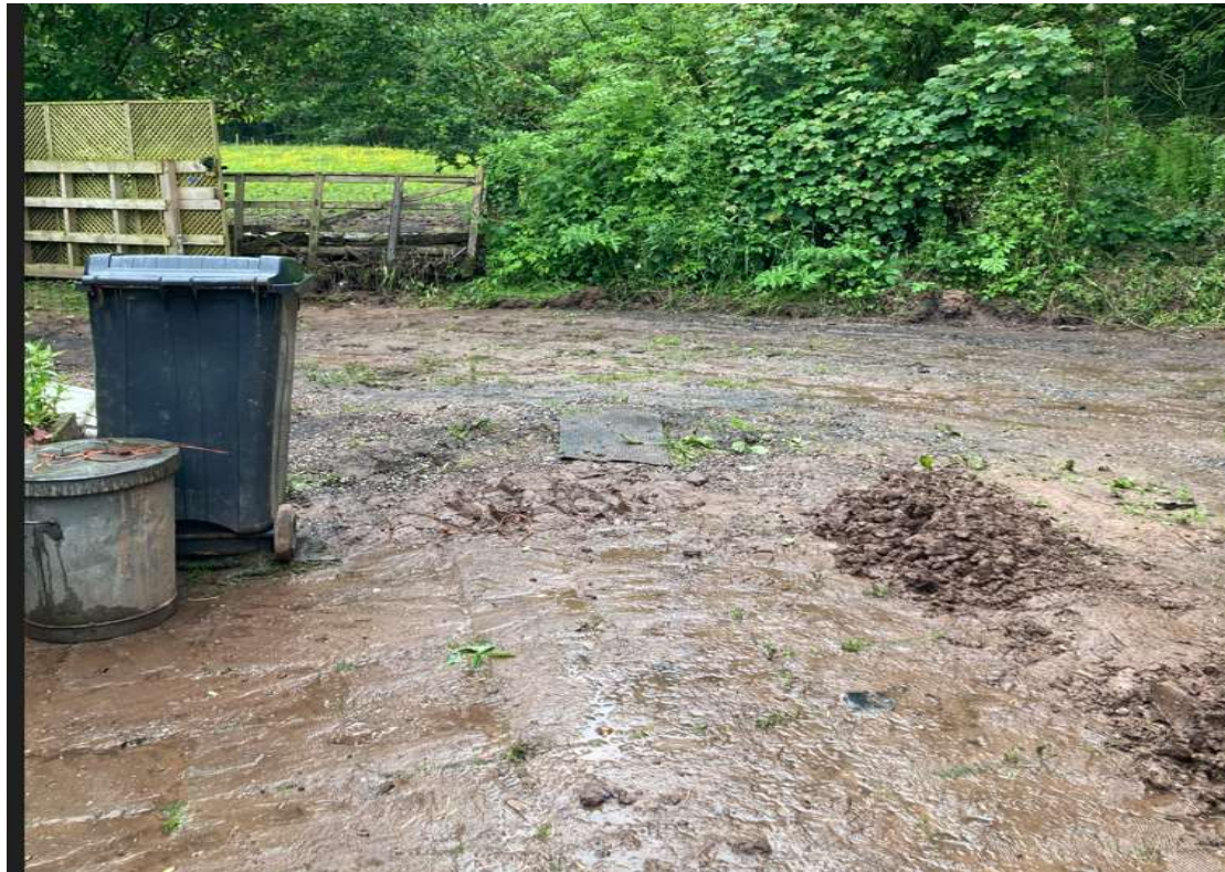
Figure 29: Field access gateway where flows exceeded from Pen Beck
