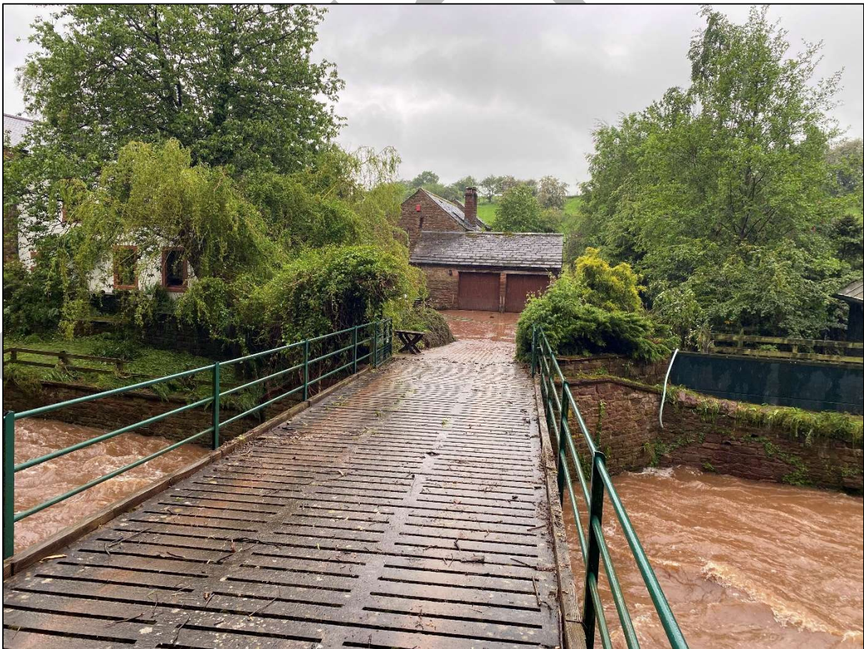
Figure 19: Access bridge to Hempgill. Flood level was above bridge deck.
