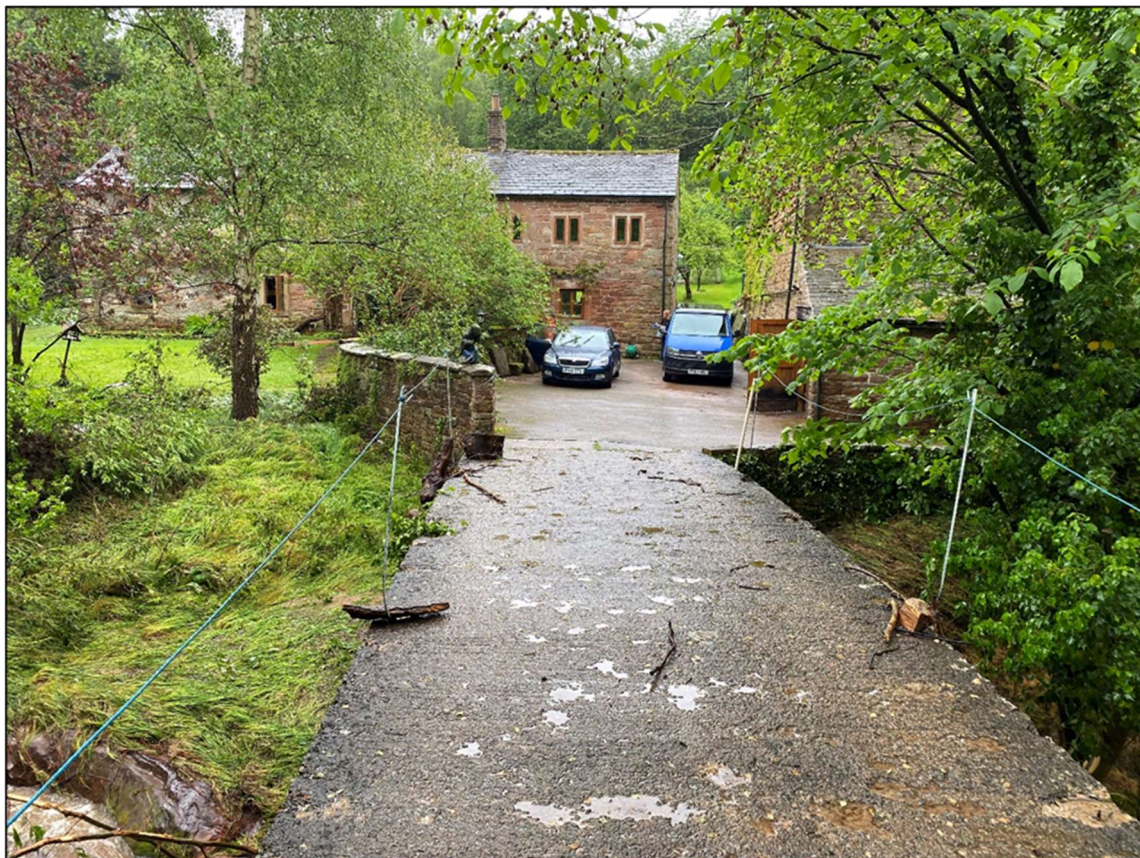
Figure 17: Bridge across Roe Beck. River flowed over the top of this bridge
