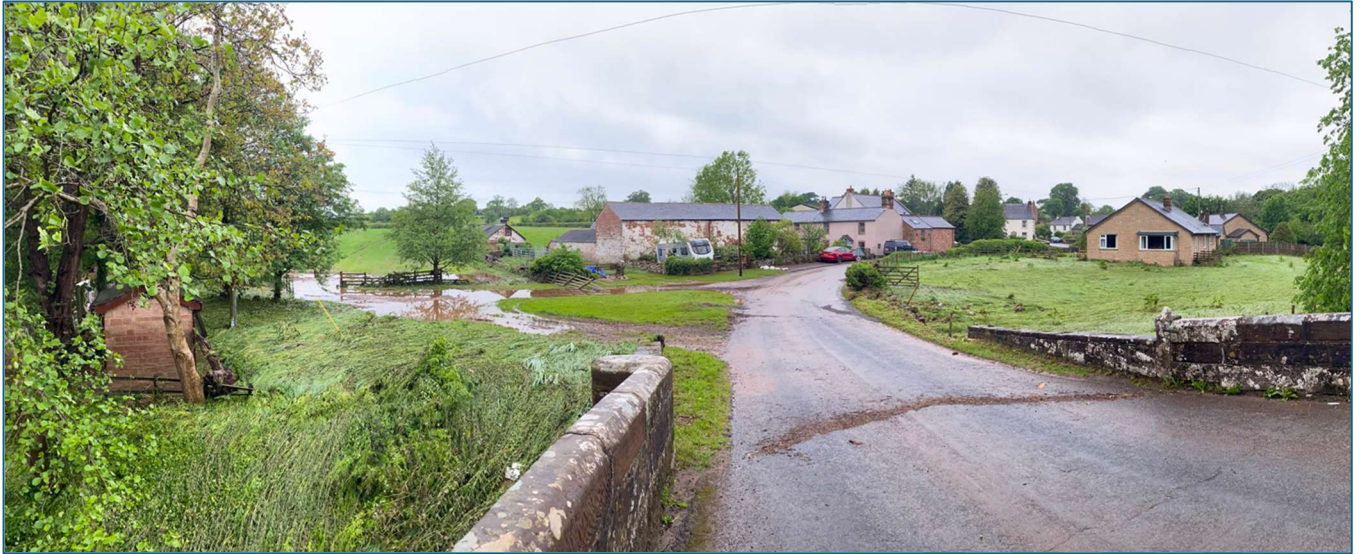
Figure 26: Looking from the main road bridge west towards Stockdalewath. High water mark on the bridge approach is visible in the foreground. Damage to field boundaries (walls and fences) on both sides of the road.
