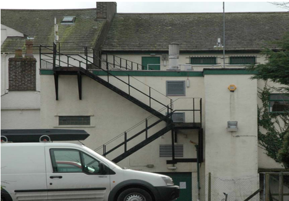
Rear extension which dominates (and obscures) original building
