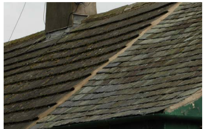
junction at the abutment of different roof coverings
