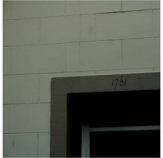
Stucco (lined out to mimic stone)
