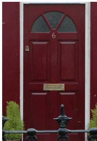
Non traditional integral fanlight. Fanlights are traditionally above the door.
