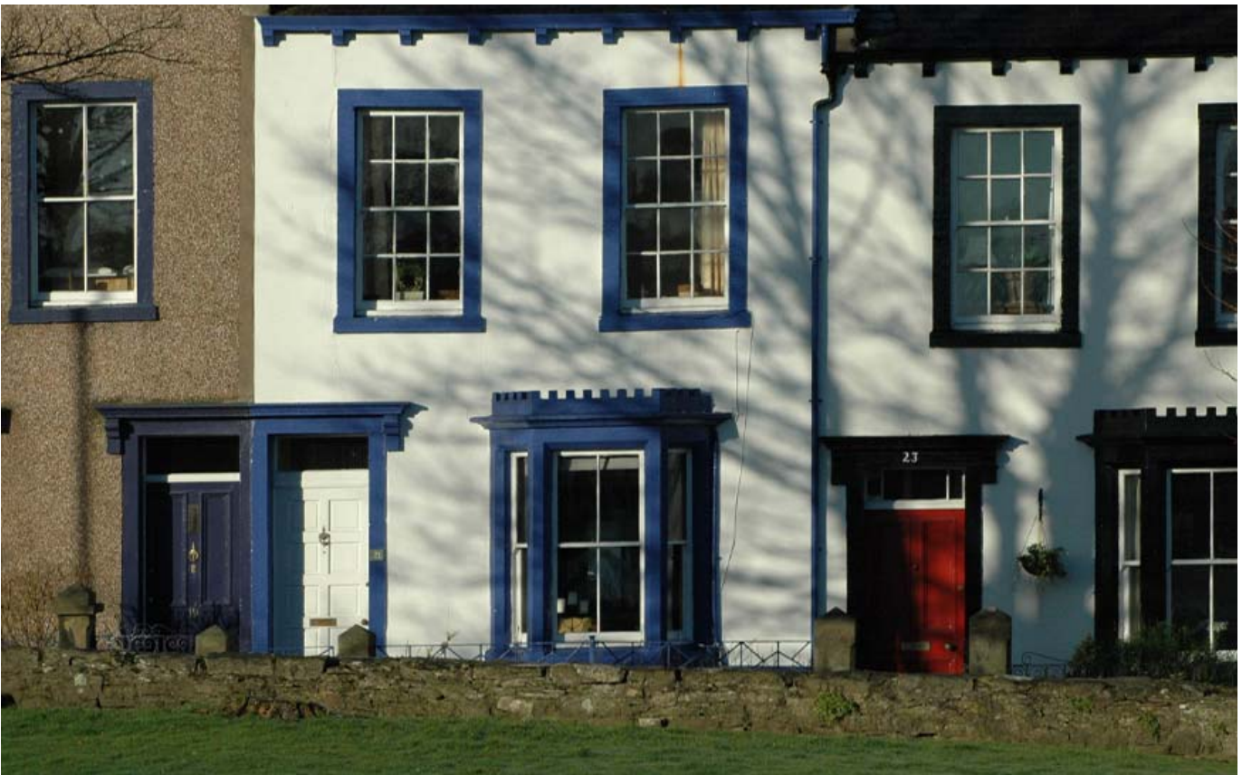
Double-hung sash windows on an early Victorian Terrace (in this case, the replacements to first floor windows are an attempt at a revival of earlier pattern)
