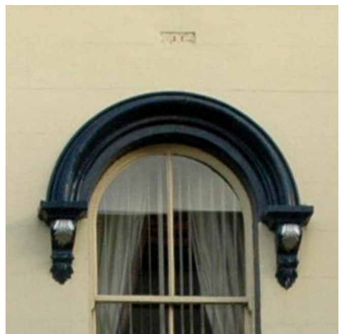
Moulded stucco window head
