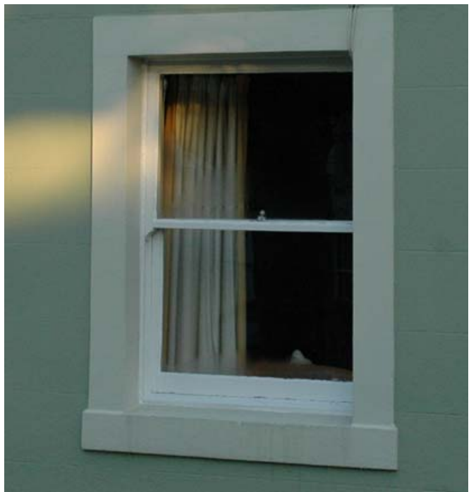
Later/modern sliding sash window, note horns to later types
