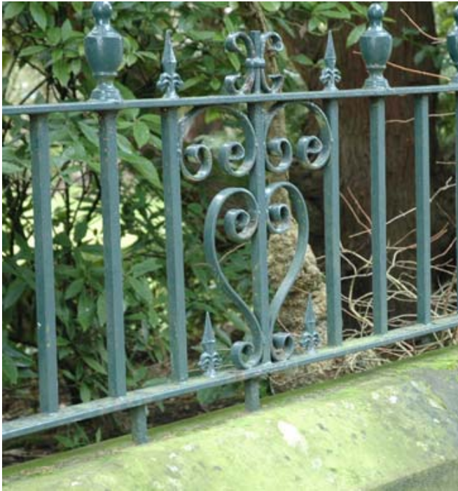
Surviving wrought iron railings
