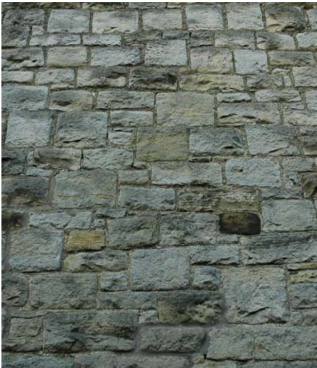
Stone laid as squared rubble
