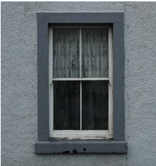
Regency-Victorian sliding sash window
