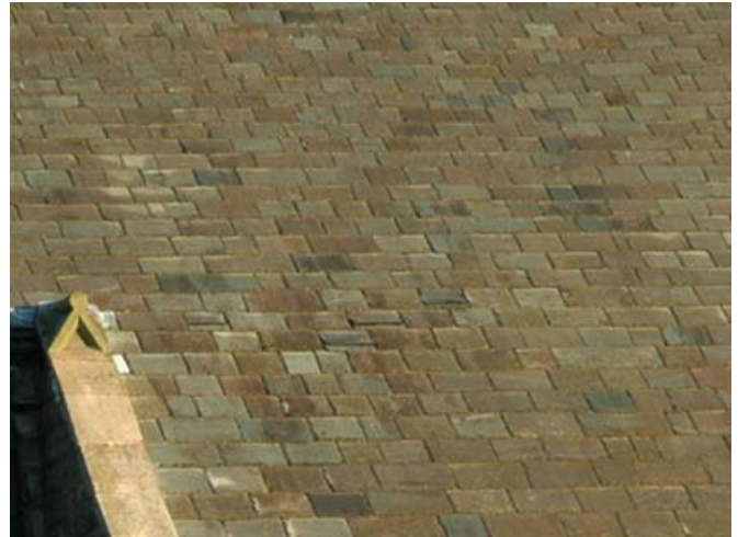
Cumbrian green slate roofing laid to diminishing courses
