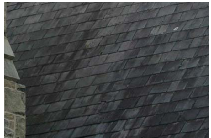
Welsh slate roofing laid to regular courses
