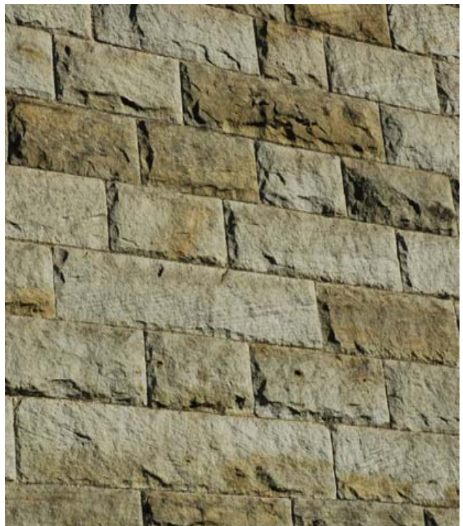
Stone laid as rock-faced ashlar
