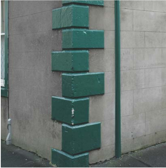
Stone dressing (quoins) to corner
